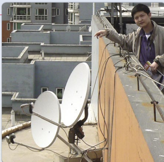
■ Additional antennas are mounted on a side railing: a 75cm dish is pointed to 134°E with a 60cm antenna motorized with a MOTECK motor.
