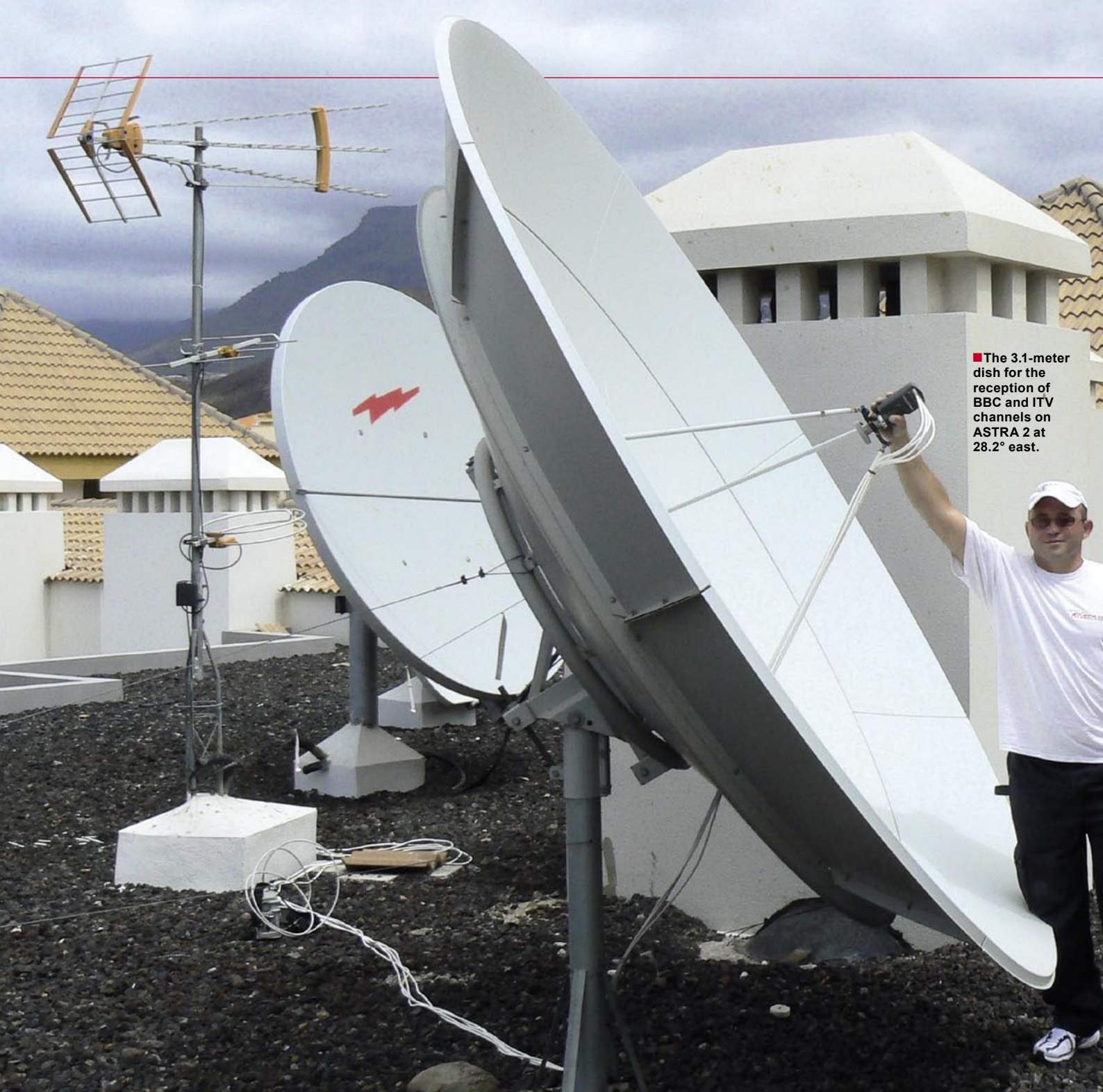
■ Diego shows us one of his tricks: the antennas are braced not only because of wind load: “This lets me easily handle fine tuning adjustments in order to precisely align the dishes.”
