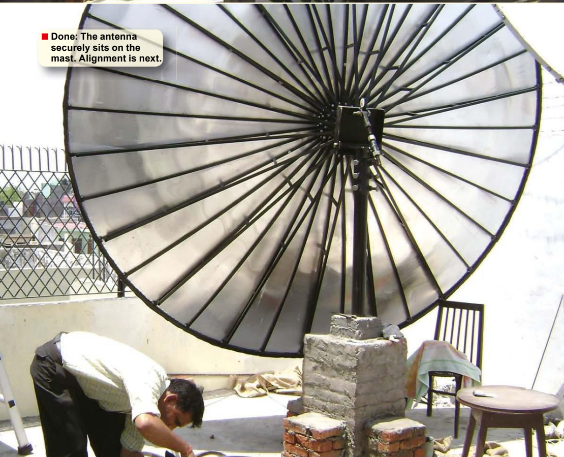
■ It took the helping hands of eight people to hoist the 2.4 m dish with its more than 200 kg onto the mast (visible in the front).
