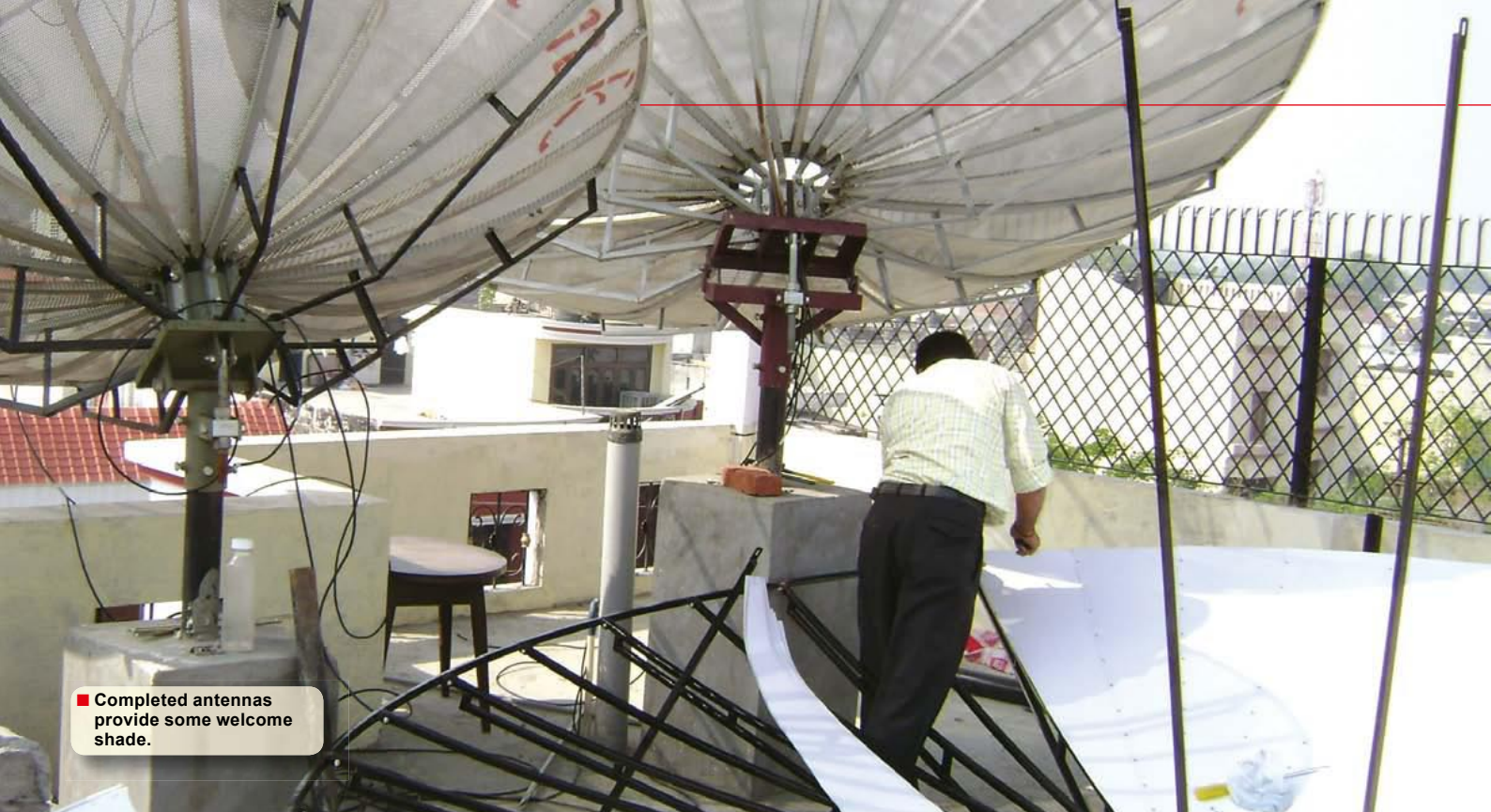
■ Screwing together the feed arms.
