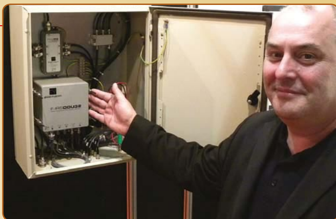
■ New at GlobalInvacom: a housing with four stacked ODU32 components that provides eight identical optical connections, capable of feeding 256 points.
