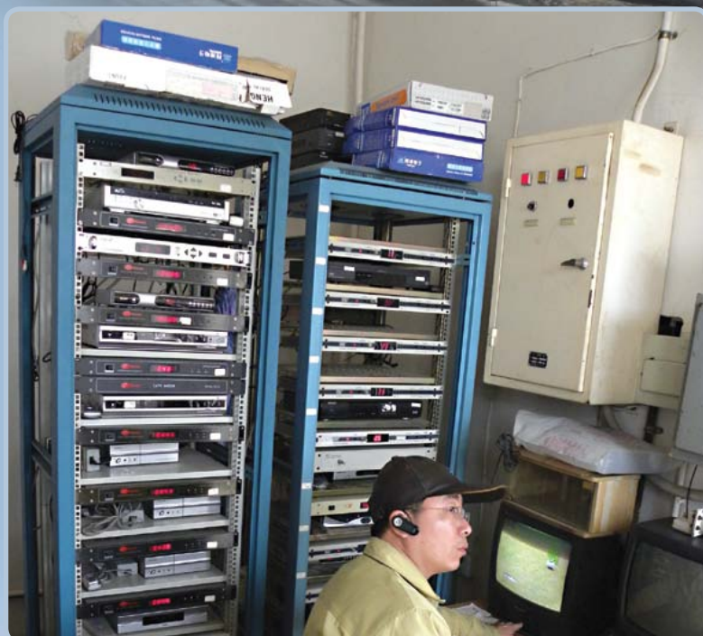
■ TV Technician Wang Yinchung set up the receivers and cable modulators in the elevator control room. He keeps an eye on reception quality with the test TVs.
